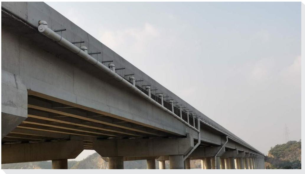
Deck runoff catchment system for preventive bridge maintenance
