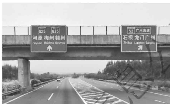
Figure 4-4 Example of exit guide sign mounted onto overpass in advance of an exit
