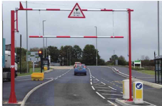
Figure 12-9 Foreign practices of height restriction warning gantry
